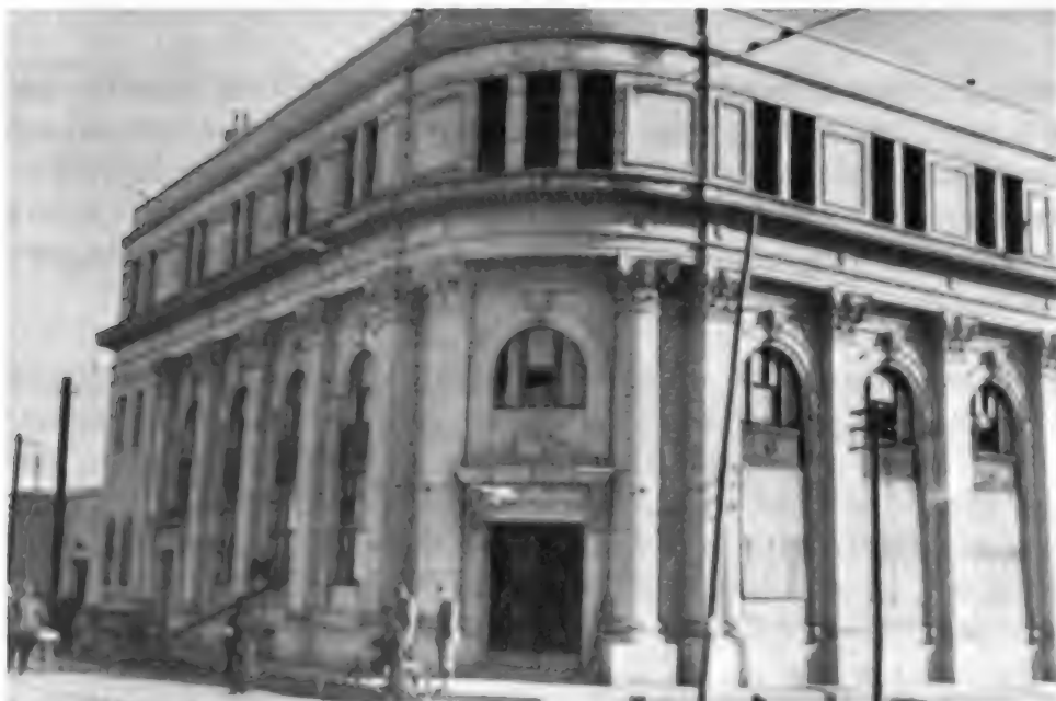
GEIBI BANK COMPANY, HIROSHIMA (BUILDING 18)
